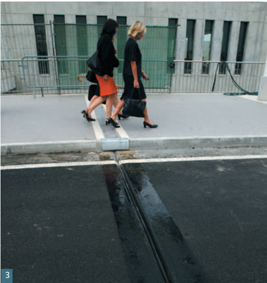
1. Anchoring a joint seam 2. 3D view of the upstand 3. JEP joint seam
