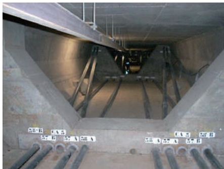
HDPE ducts for external prestressing
