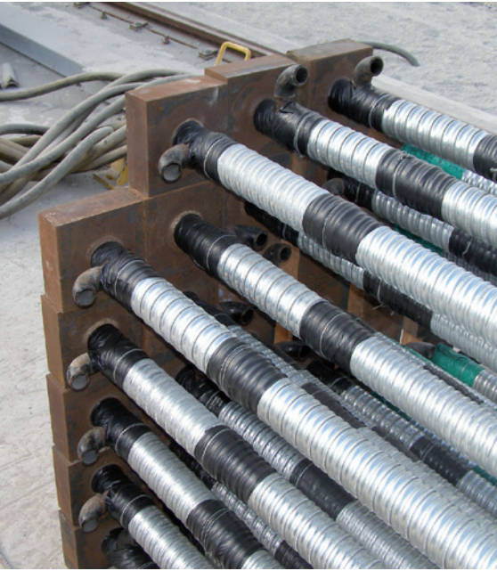
Prefabricated bar tendons
