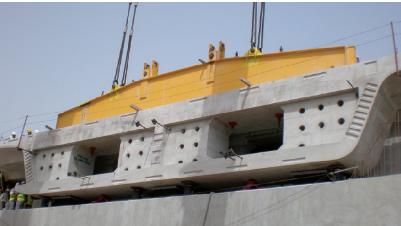
Lifting : prestressed connection between a segment and a beam.
