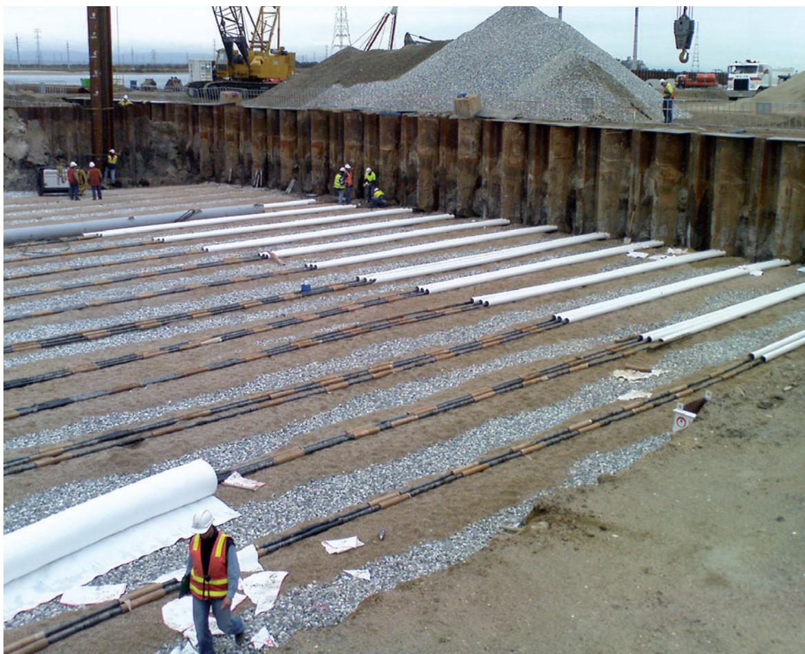
Permanent ties for quay walls
