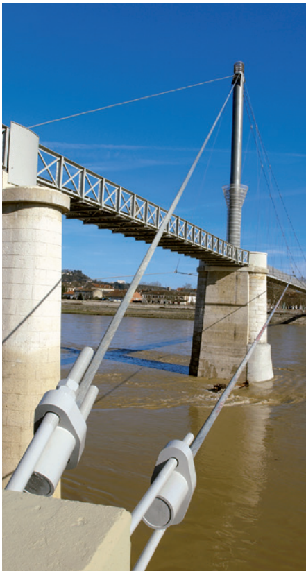
Anchorage of steel ropes
