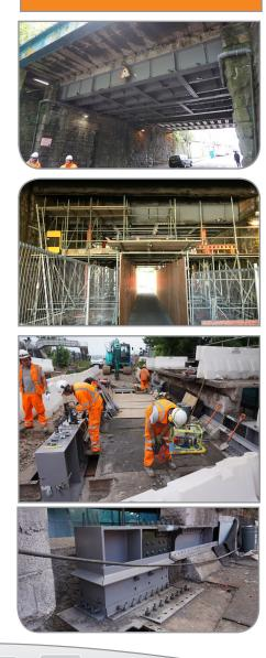
Freyssinet was chosen to work for Taylor Woodrow on St Marks Bridge off the back of successfully completing Muller Road bridge. Both structures had a similar scope – jack the steel deck then cut off and replace the corroded ends of the main girders. However, as the design delivery had been outside of Freyssinet's control on Muller Road, and there had been delivery and clash problems, Taylor Woodrow awarded an advance contract to Freyssinet to do the temporary works design.
