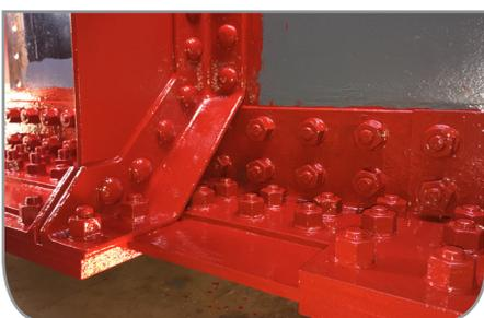
During the earlier refurbishment of Muller Road rail bridge, the ends of the main girders were found to have serious local corrosion where the bridge sat on the abutment. Before being brought back into use as part of Bristol's Filton Bank four tracking project, it was necessary to restore full strength. Principal Contractor, Taylor Woodrow, appointed Freyssinet to do this work in July 2017.
