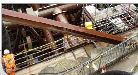
The work on Farringdon Station involved the installation and stressing, in a complex sequence, of 75 number reference 60 flat jacks (600mm diameter) and two number Enerpac 8002 pot jacks in order to de-stress basement props in a controlled manner.
