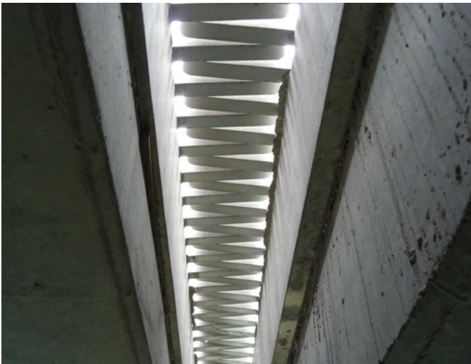
WP joint seen from below
