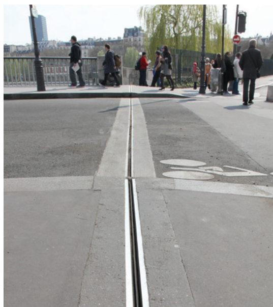
WR 50 joint Île Saint Louis bridge - Paris
