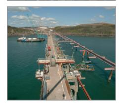
The existing jetty is 1km long, comprising 125 separate support structures. The jetty head is a further 1km in length and comprises 5 existing berths that will be converted into 2 LNG super tanker berths.
