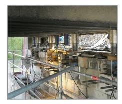
Valenton Rail Bridge allows the Great Belt Line, which diverts TGVs and freight around Paris, to cross the tracks of Villeneuve yard, in the Val de Marne, south-east of Paris. To allow track improvements in the area, and to permit the passage of a new type of larger rail carriage, the Valenton bridge had to be lifted by 400mm.
