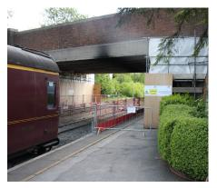
Butterley Station overbridge has a 15m span deck with eight riveted steel girders spanning onto concrete abutments.
