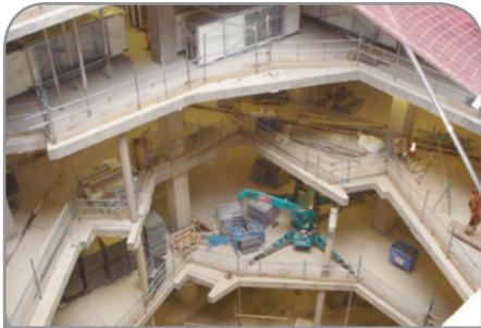
Each floor plate was divided into four pours approximately 30 by 24m. Infill strips were used between some pours to provide temporary releases to the restraint to slab shortening that the RC cores would otherwise have offered. The structural grid was typically 8 by 8m but spans were substantially longer at the irregular slab edge at the courtyard. The slab was also asked to cantilever up to 3.5m in some areas of the courtyard. The PT slabs were generally 225 or 250mm thick.
