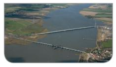
The 1.2km long structure has 26 spans installed by incremental launching and weighs more than 22,000 tonnes. The construction of each 45m span was typically completed in 8 days instead of the original 10 days expected in planning, with the final span being launched in February 2008
