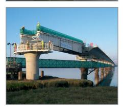
The launching cables had no profile and were grouted using Freyssinet's high speed grouting technique where the grout is injected to maintain a minimum flow of 20m per minute. This was verified by undertaking a full scale grout trial on the job.
