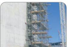
The post tensioning system for each tank comprises of 70 No "hoops" with each "hoop" comprising of 2 19C15 tendons installed in the form of horizontal tendons only stressed at buttresses located at 90 degree apart.
