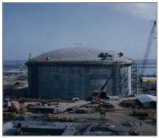
Following the successful completion of the post tensioning to two 130,000cum LNG tanks for the Atlantic LNG Project at Point Fortin in Trinidad and Tobago. Freyssinet Ltd were awarded the sub contract for the supply and installation of the post tensioning system to the third tank of 160,000 com capacity on the same site.
