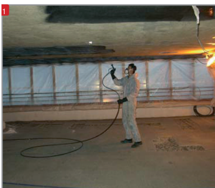
1 Application of conductive coating anode system
