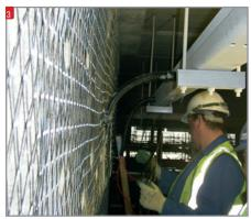
Freyssinet undertook surveys of the sub-structure after the dock was pumped dry to assess the condition of the concrete particularly in relation to corrosion damage caused by ingress of chlorides from the saline dock water.
