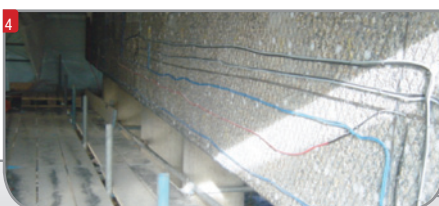
3 Pier showing initial stages of CP System
