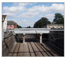
The Stratton Street Bridge carries Biggleswade High Street over the East Coast Main Line. The deck had life-expired but the substructures could be retained with some strengthening.
