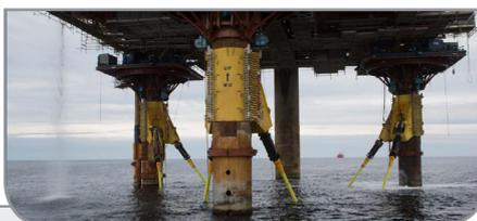
The Siri oil platform is a production jack-up, anchored in the North Sea 220km off the coast of Denmark. In 2009, an detected cracks in the support structure and unsatisfactory fatigue life in the legs where they were connected into the base on the seabed.
