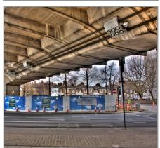
Hammersmith Flyover is an elevated roadway in West London which carries the A4 dual carriageway over the central Hammersmith gyratory system. Completed in 1961, it is one of the first examples of an elevated road constructed using reinforced concrete.
