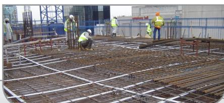
The Library of Birmingham was originally conceived as a structural steel frame. During the tender period, and in order to realise the full value engineering benefits, the frame was changed to RC with post-tensioned slabs and beams.
