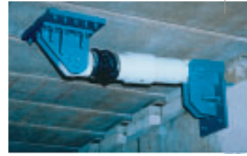
Placing on the pier head in the context of retrofitting (Hambrook bridge, UK)
