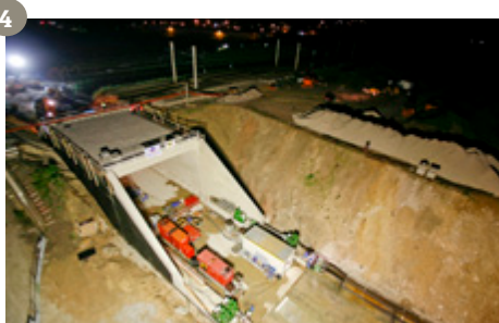
4 - Final sliding and backfilling
