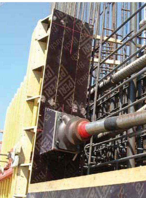
structure. Sheath thickness is chosen depending on the lateral pressure exerted in the curved sections and the movement of the strands during tensioning.
