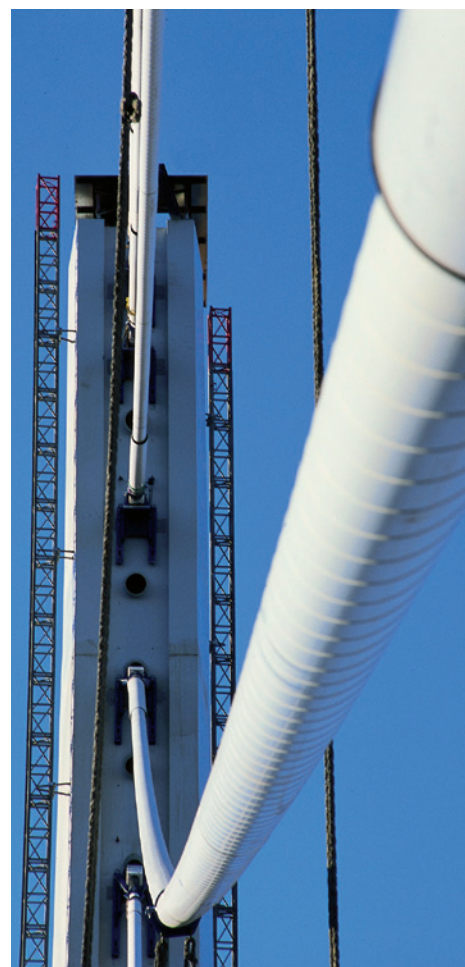
Helical fillet Millau bridge / France
