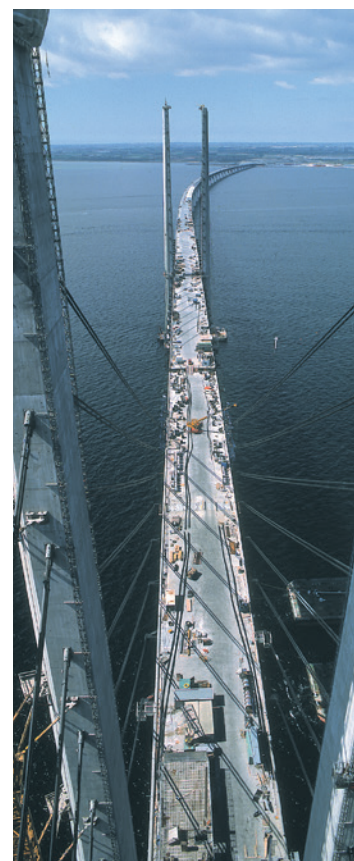
Øresund bridge Denmark-Sweden
