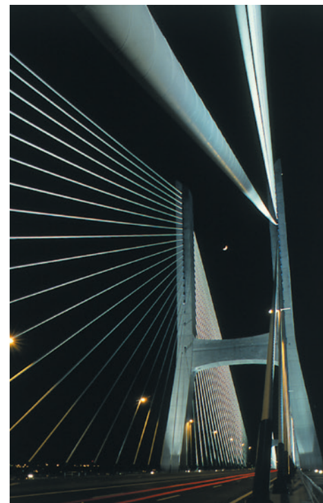
Light fittings Vasco de Gama bridge / Portugal
