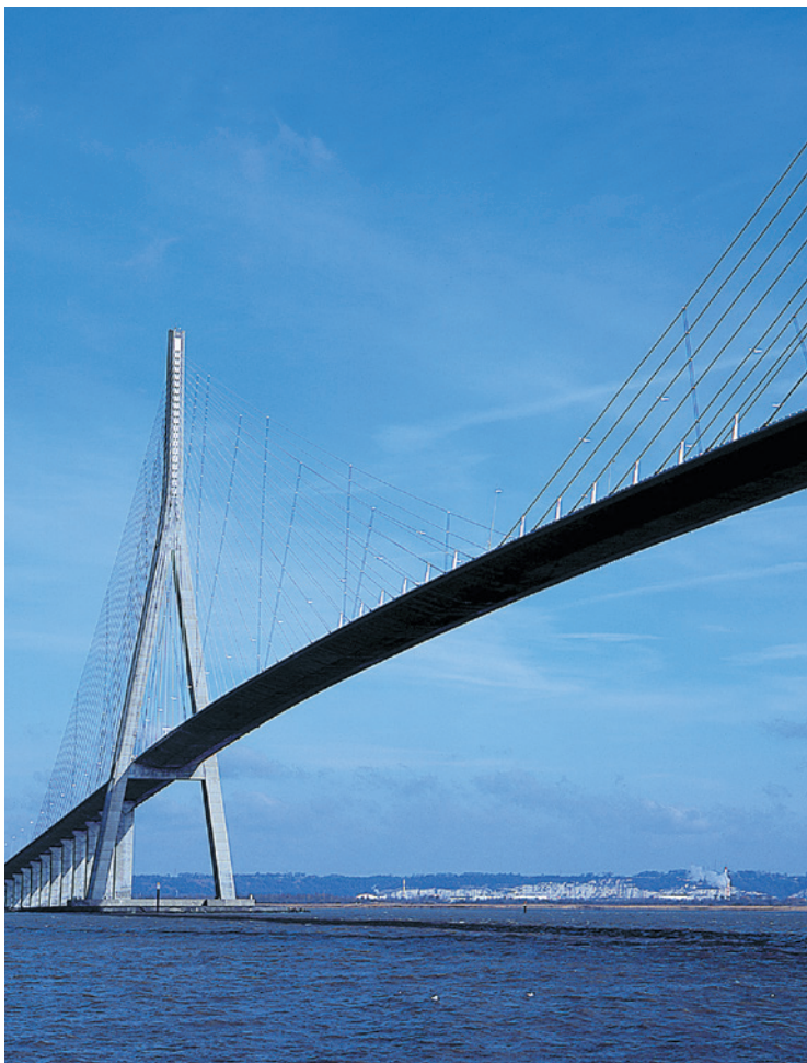
Normandie bridge cross tie / France
