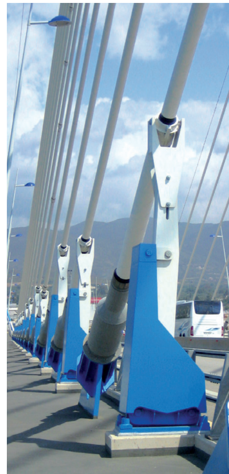
PED damper Charilaos Trikoupis bridge / Greece
