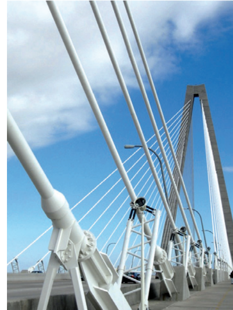
FED damper Cooper bridge / USA
