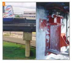
Gatwick's elevated transit system carries two automated passenger tram cars between the north and south airport terminals on a viaduct. The structure crosses the A23 dual carriageway in the form of an 82 m long, two span, continuous box beam with cantilevered outrigger track supports. The structure is supported on two bearings at each verge abutment and on a central supporting column.
