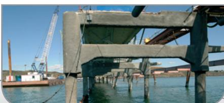
The existing jetty is 1km long, comprising 125 separate support structures. The jetty head is a further 1km in length and comprises 5 existing berths that will be converted into 2 LNG super tanker berths.
