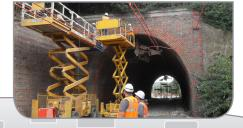
Harfleur Tunnel is located on the Paris to Le Havre line in Northern France between Harfleur and Havre-Granville Stations. It is 48m long, 8m wide, 6m high and curved on a 1200mm radius. Two personnel protection refuges exist on each side.
