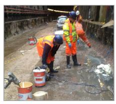
Freyssinet was appointed by Bachy Soletanche to carry out PU resin injection to 2no. one metre deep concrete invert approach ramps to Connaught Tunnel. The tunnel was built in 1878 and is situated on the formerWoolwich branch of the North London Railway, running under the Royal Docks and City Airport in London
