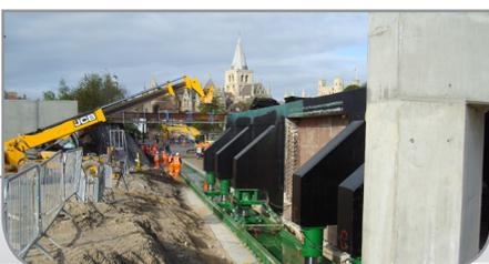
Freyssinet's Autoripage® technique is used when a structure is built to one side of the track. When the rail blockade has been secured, the track and embankment are removed and the newly exposed ground is levelled. The structure is then slid from its constructed position beside the tracks to its final position.
