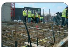
Numerous penetrations have been accommodated in the design – from temporary openings for hoists, 4.6m long slots for risers and edge fixings for climbing edge-protection screens.
