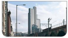
The structure consists of 35 levels, all formed from post-tensioned concrete. The thinness of the slabs allows extra storeys to be squeezed in for a set building height, which can really make a difference to the financial viability of tall buildings.
