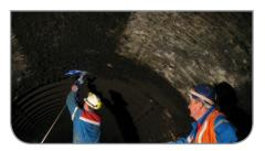
The £250,000 contract awarded to Freyssinet Makers involved the injection of over 60 tonnes of cementitious grout and 3000 litres of polyurethane resin to fill out and waterseal the voids in the tunnel lining between the Buchanan Street and St Enoch's stations.
