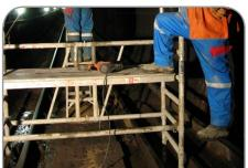
Extensive monitoring of the tunnel took place during the works to ensure the integrity of the tunnel linings while the works were carried out during nightshift possessions of the track.
