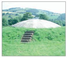
Upper Keel service reservoir forms part of the STW drinking water distribution network in the Welshpool area of Powys. Freyssinet were contracted by Black and Veatch to undertake structural repairs and waterproofing works to the service reservoir as part of the Severn Trent Water AMP 4 contract. The reservoir is of in-situ concrete construction. The base and walls are buried and the domed roof is exposed.
